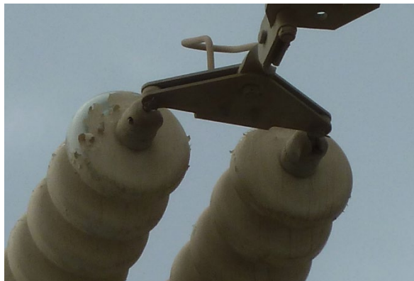
Figure 10: Example of poor adherence resulting from poor application on site and lack of cleanliness
