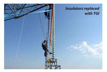
Toughened glass has an extremely high impact strength making it difficult to break. If it does break, the outer shell falls away completely in small kernel size pieces (like safety glass).
