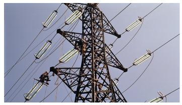
Suspension and tension insulators for transmission and distribution lines (from 15 up to 1,000 KV) with mechanical load from **40 kN** to **840 kN** in both standard and fog type profiles as well as open profile for desert environment
