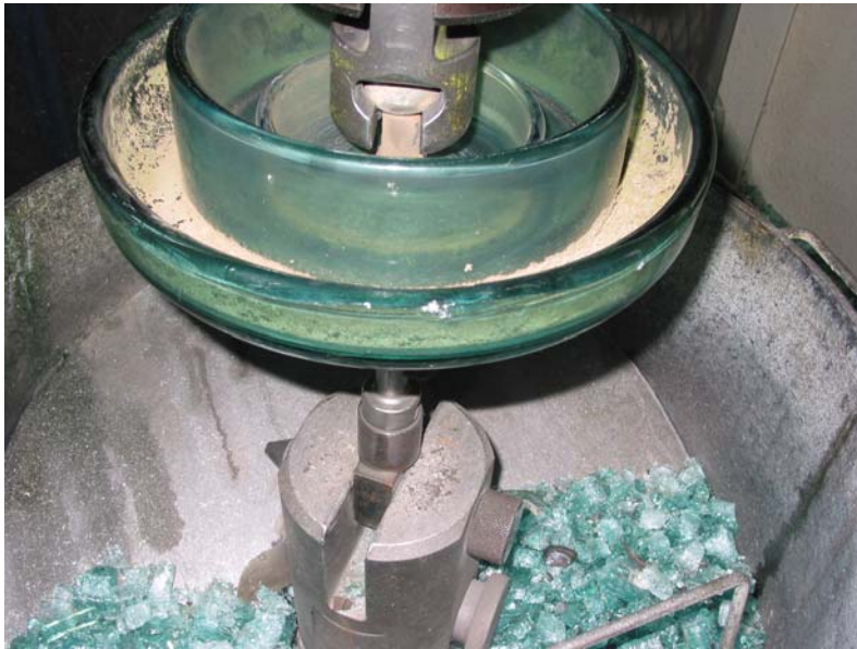
Figure 19: Itaipu insulator during the mechanical test (polarity (-))
