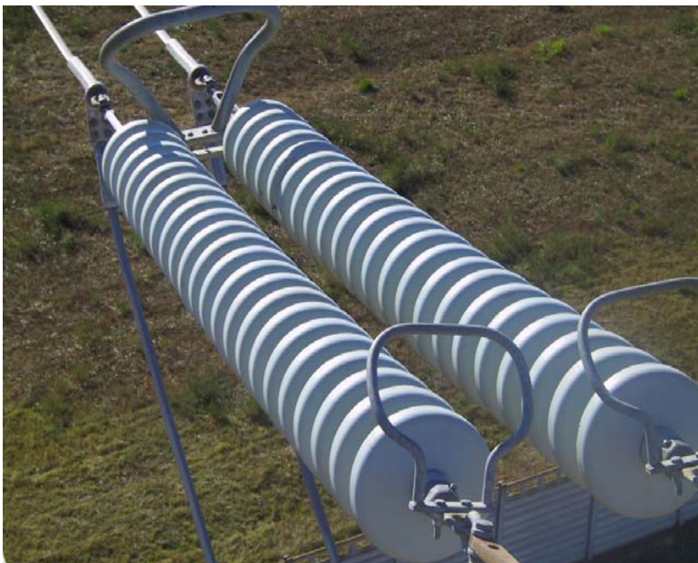
Coated anchor strings installed on a 380 kV line in the proximity of the Mediterranean coast, North of Rome. Minor scratches produced during the installation may be noticed.
