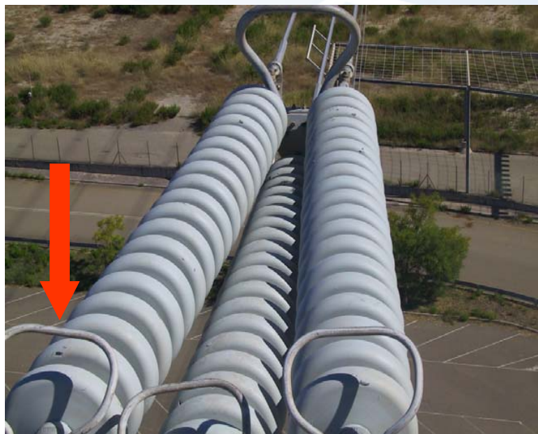
Coated anchor strings installed on a 380 kV line in the proximity of the Mediterranean coast, North of Rome. Minor scratches produced during the installation may be noticed.
