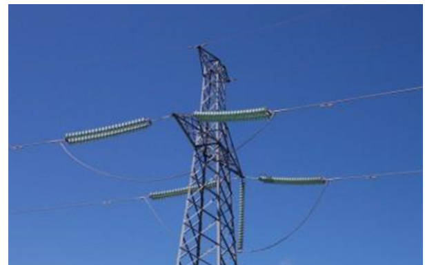
Figure 8 Silicone coated toughened glass insulators installed in Italy on the Terna 200kV dc line
