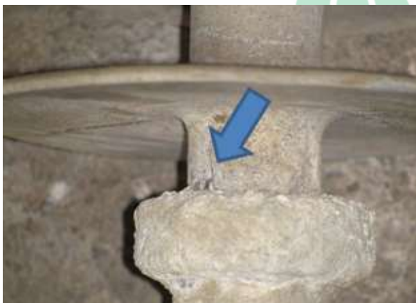
Figure 3: erosion at the shank of a silicone insulator returned from a DC line
