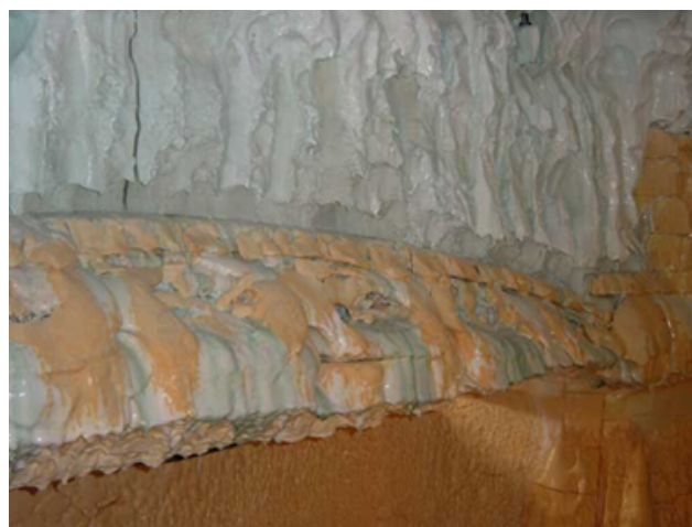
Figure 4: Typical aspect of the inner walls of a glass furnace after several years of service
