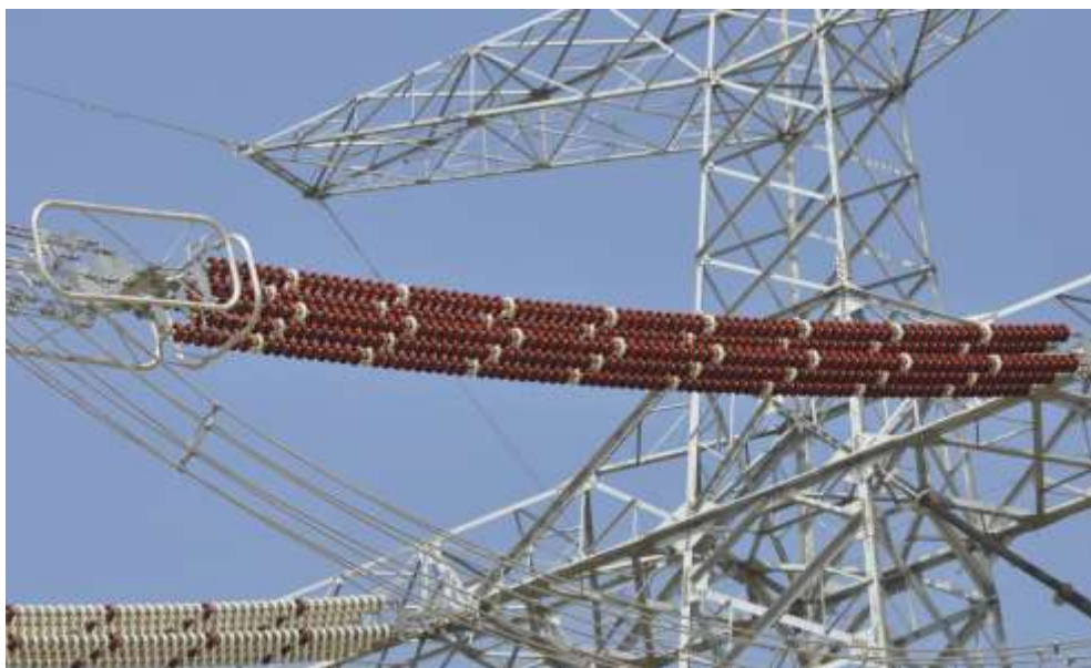
Figure 12: Tension strings of the Inner Mongolia 800kV HVDC line with red and white coloured coatings over toughened glass insulators
