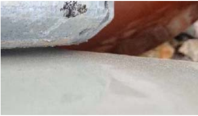
Figure 7. Typical gap between the cap and the dielectric in porcelain designs
