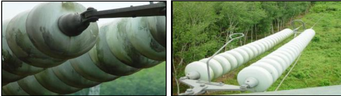
Figure 4: Difference of pollution between polarities on a 350kV DC line (left +, right -).
