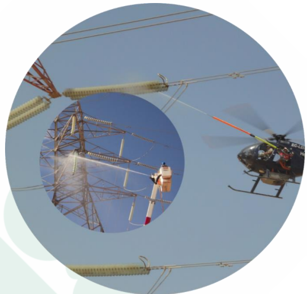
Figure 5: Overhead line cleaning operations
