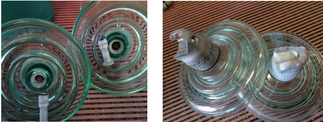
Figure 17 : Typical aspect of the glass units after the test
