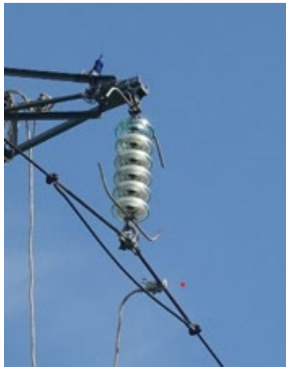
Figure 8: Example of smart insulator 3S with typical reading and analysed response
