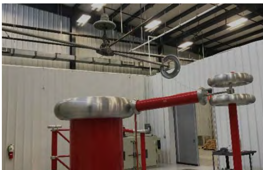
Figure 6: Power frequency verification prior to implementation of an investigation program
